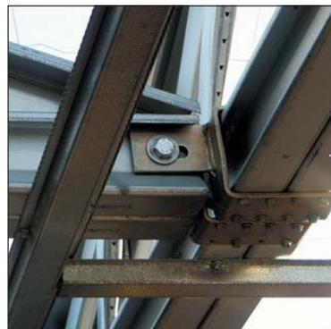
Relatively sophisticated joints can be overcome by incorporating heavier guage steel, hot dip galvanized for corrosion protection.
