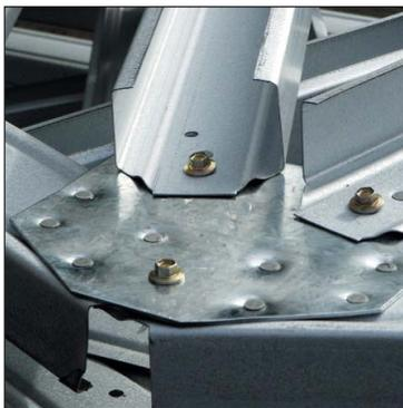
Typical construction joint.
